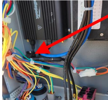
Relay location for ECU power and Crank
